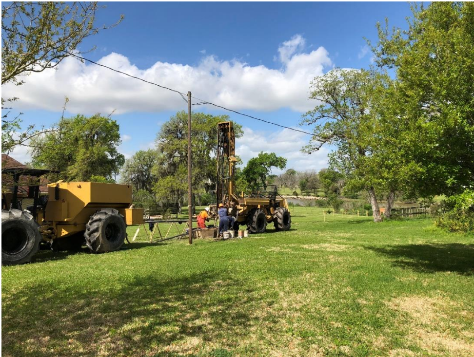
geotechnical bores safely completed at Slap Out Gully on March 23, 2018
